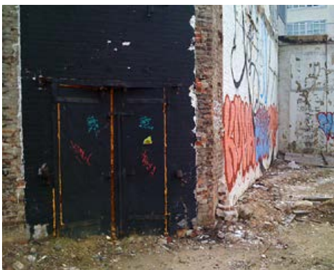
Portal location by day, Queens, 2011
